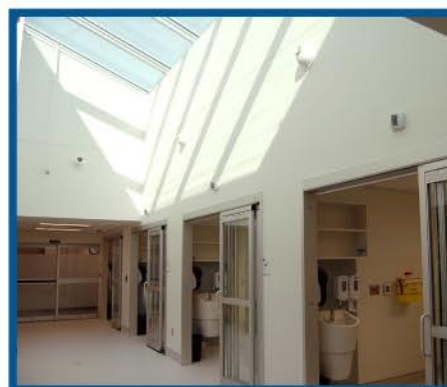
The OR preparation area can be found in what was HGH's courtyard space. A beautiful skylight was installed to bring light into the department and each preparation room is private the best patient care and comfort in advance of a procedure.
